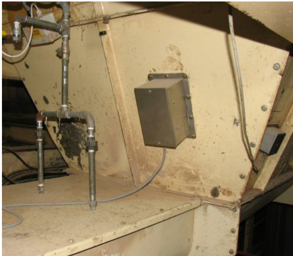
The moisture meter and water addition pipes
